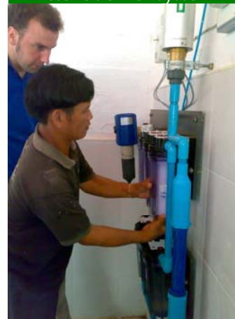
Figure 11 Training and installation of system
