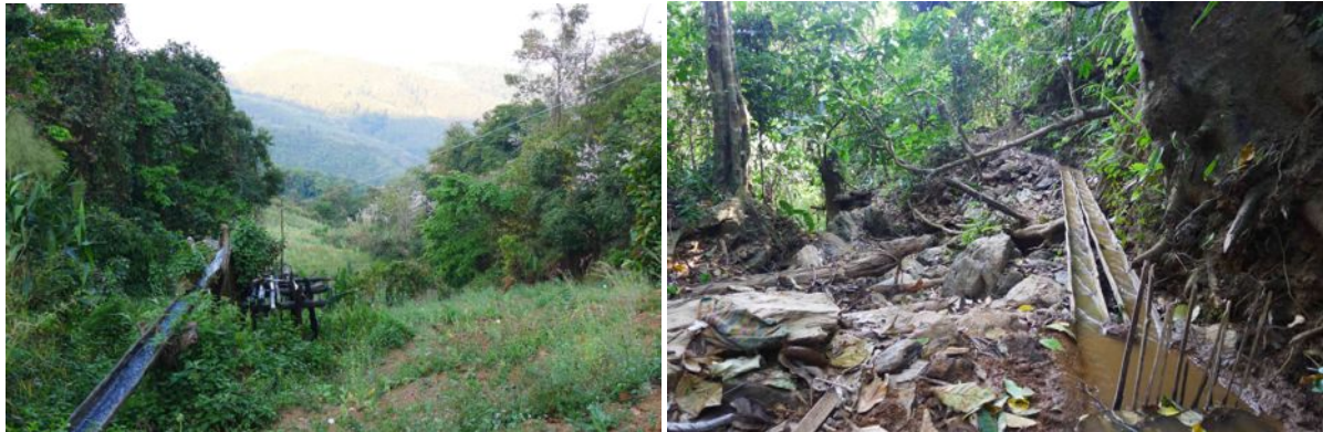
System at Aiseng (left) and canal at Chakhansene (right)
